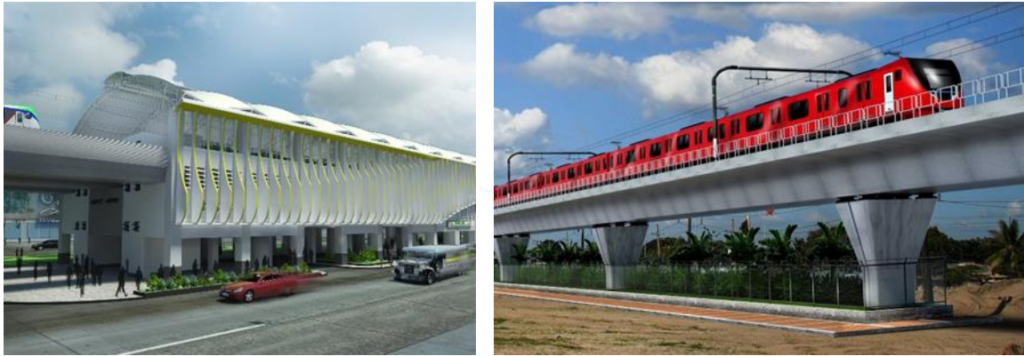
External View of North-South Commuter Railway (Image)
